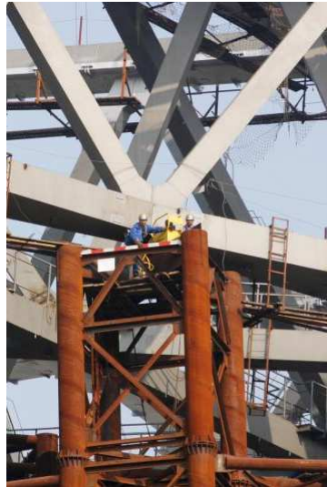
remove scaffolding / temporary bracings
